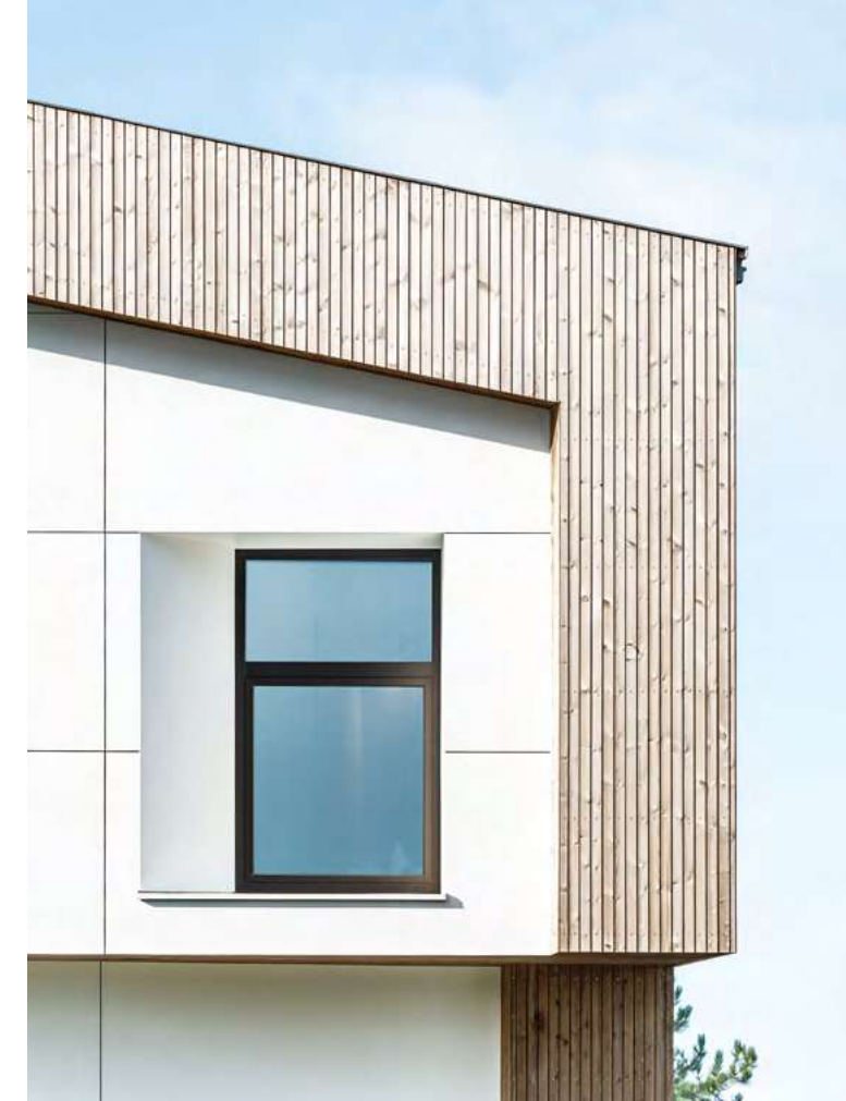
Invisible mounting with the Swisspearl Sigma 8 Pro system
