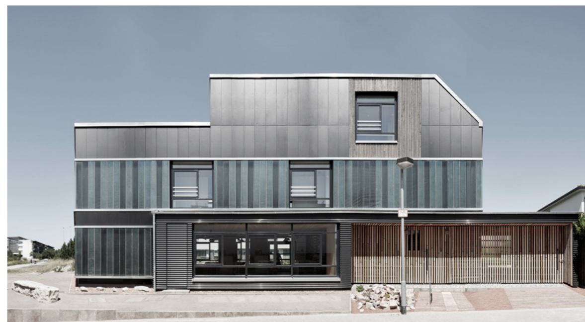
... and reused for the cladding of a (90% recycled) home.
