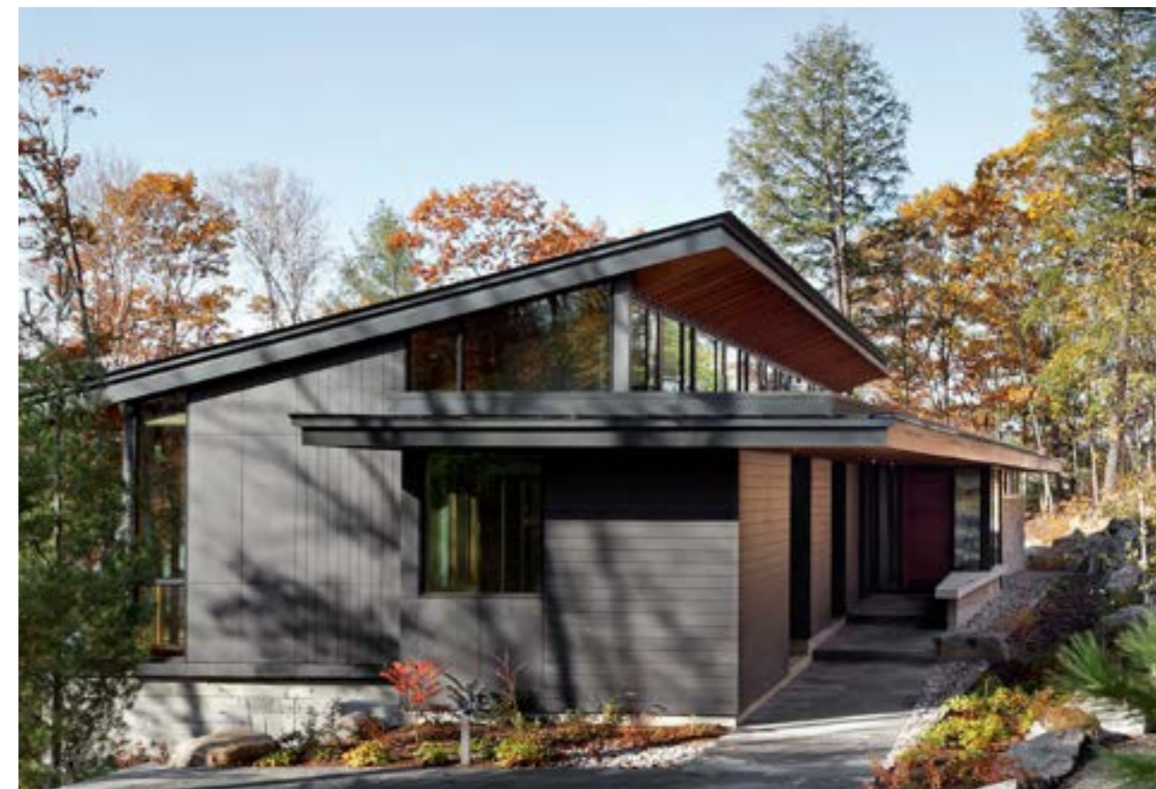
House on Haliburton Lake, Ontario, Canada. Architect: +VG, Toronto, Canada. Photographer: David Whittaker Photographer Inc., Toronto, Canada.
