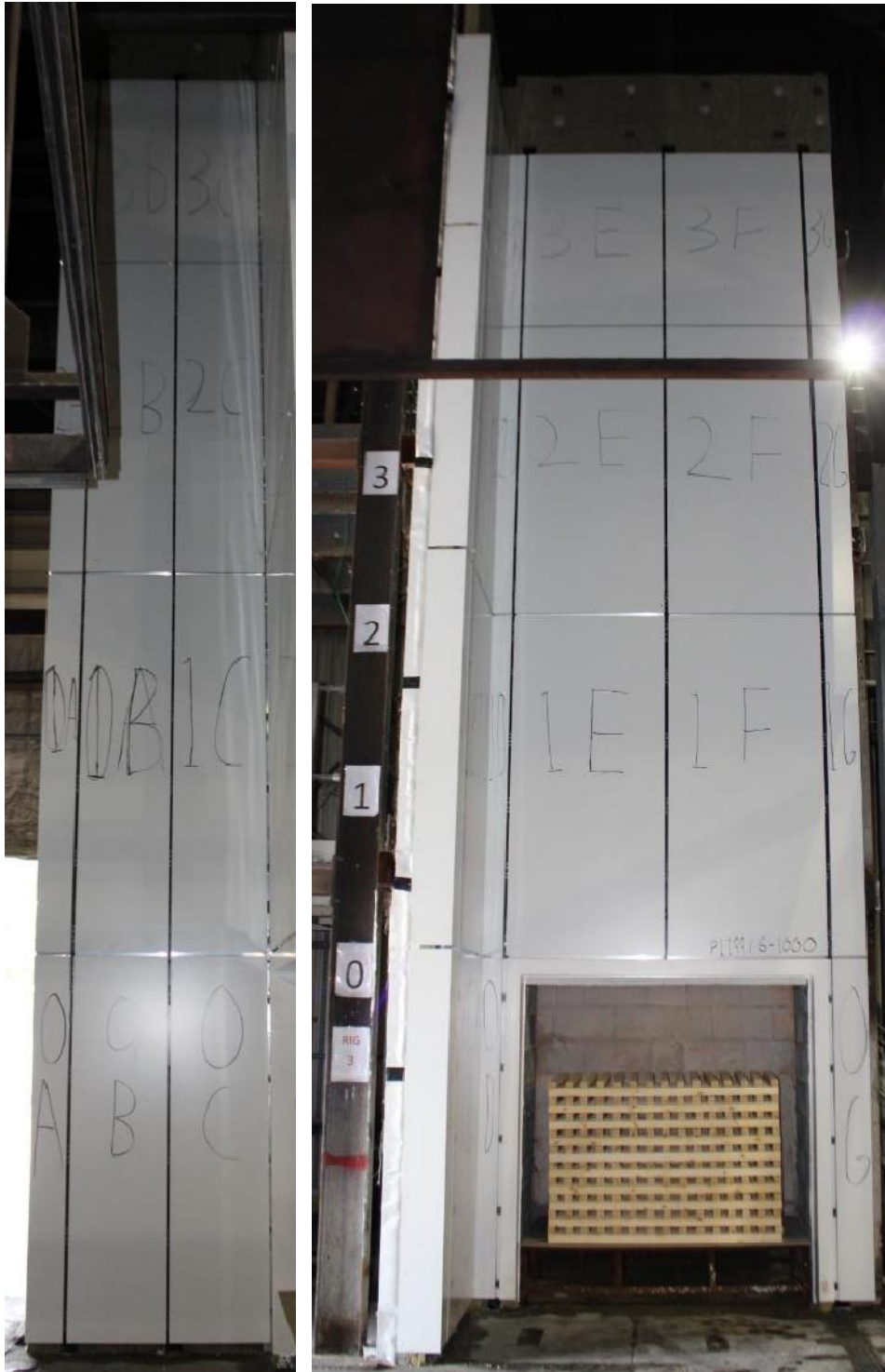
Figure 2. Completed installation prior to test.
