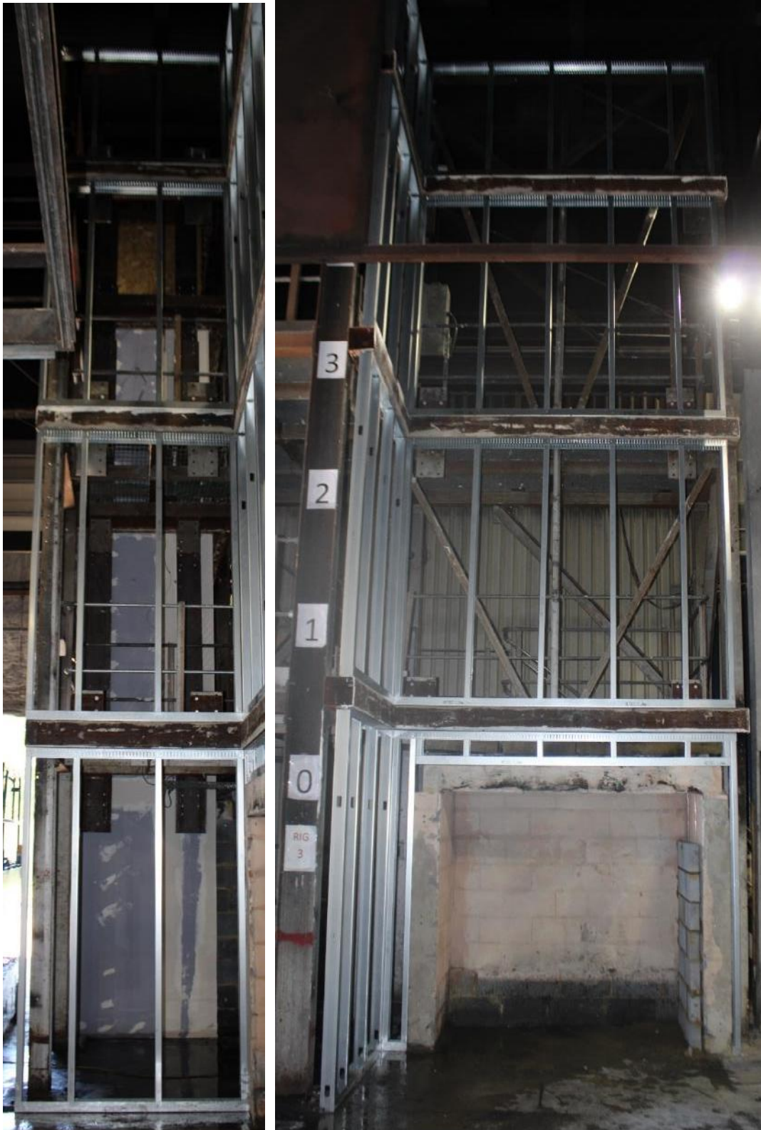
Figure 2. Installation of steel framing system (SFS).
