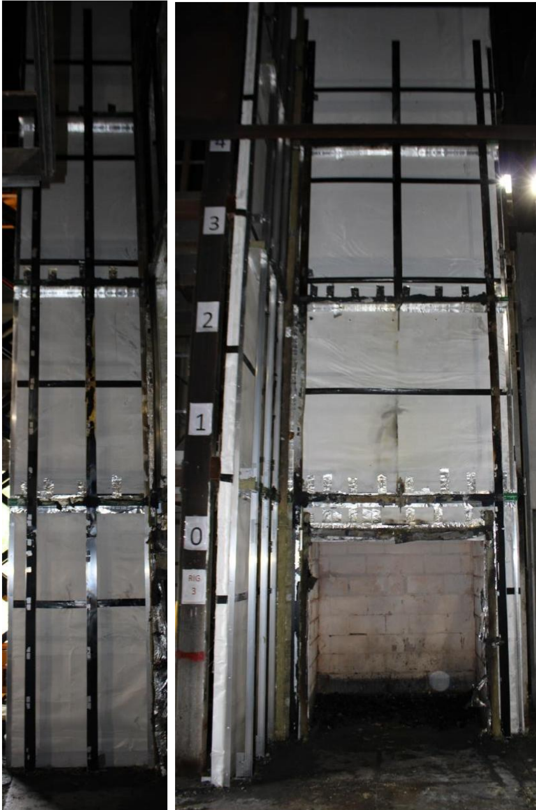
Figure 54. Full-height photograph following removal of insulation.
