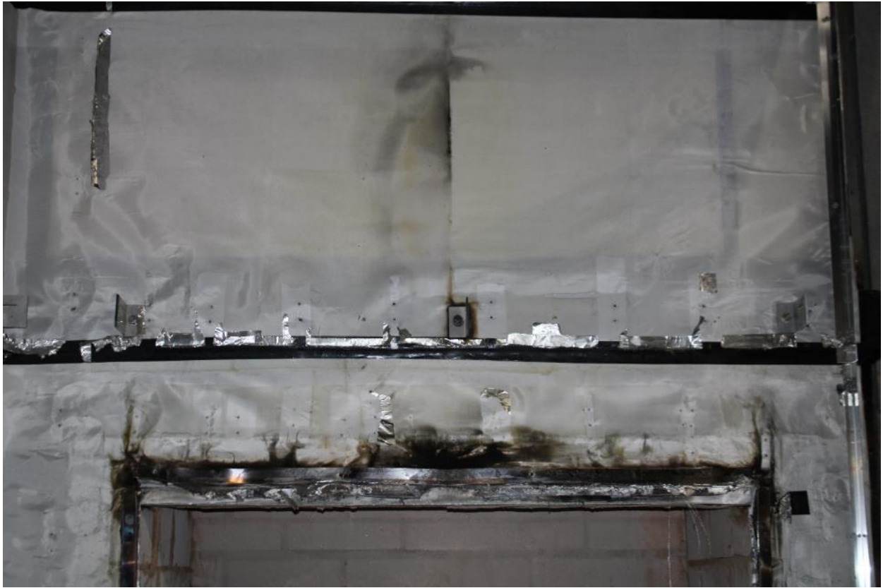
Figure 62. Close up photograph of breather membrane and brackets.
