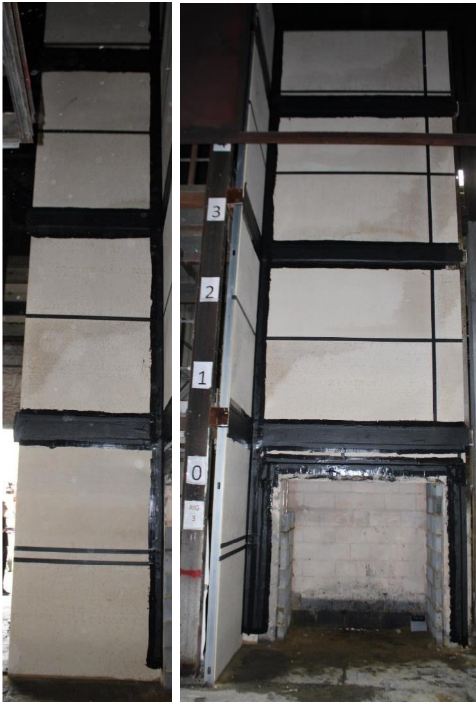
Figure 6. Installation of EPDM membrane.
