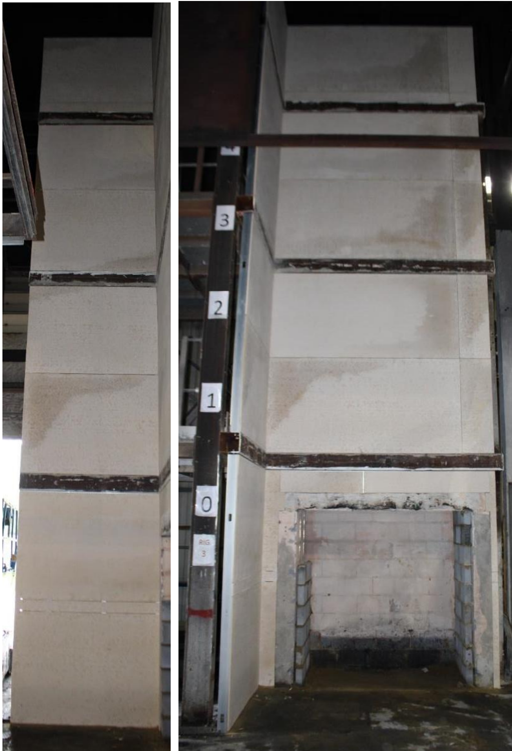
Figure 5. Installation of sheathing board.
