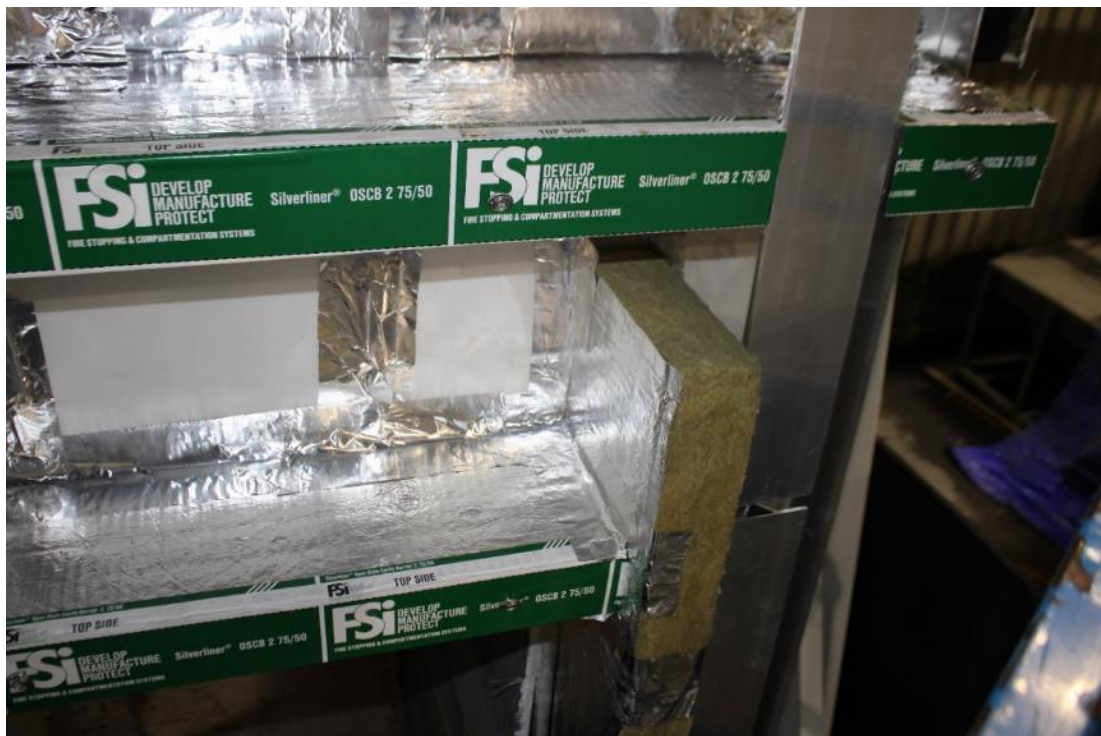
Figure 17. Horizontal and vertical barrier joint.
