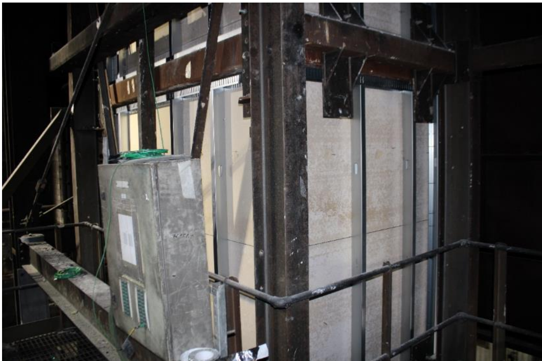
Figure 65. Sheathing board at rear of system at level 2.
