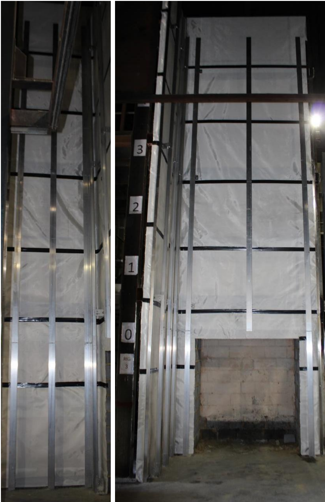
Figure 8. Installation of brackets and profiled 'T'-shaped rails.
