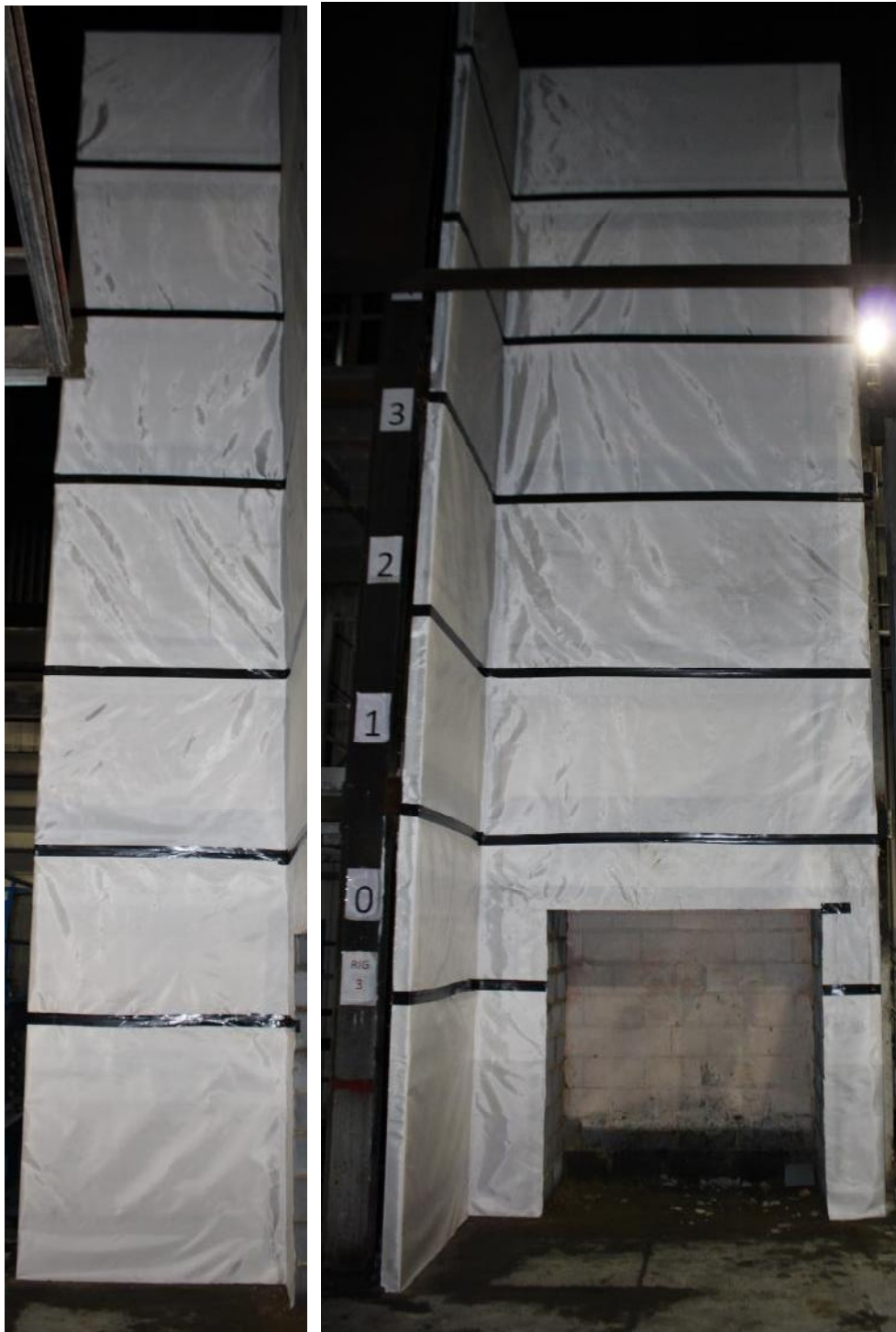
Figure 7. Installation of the breather membrane.
