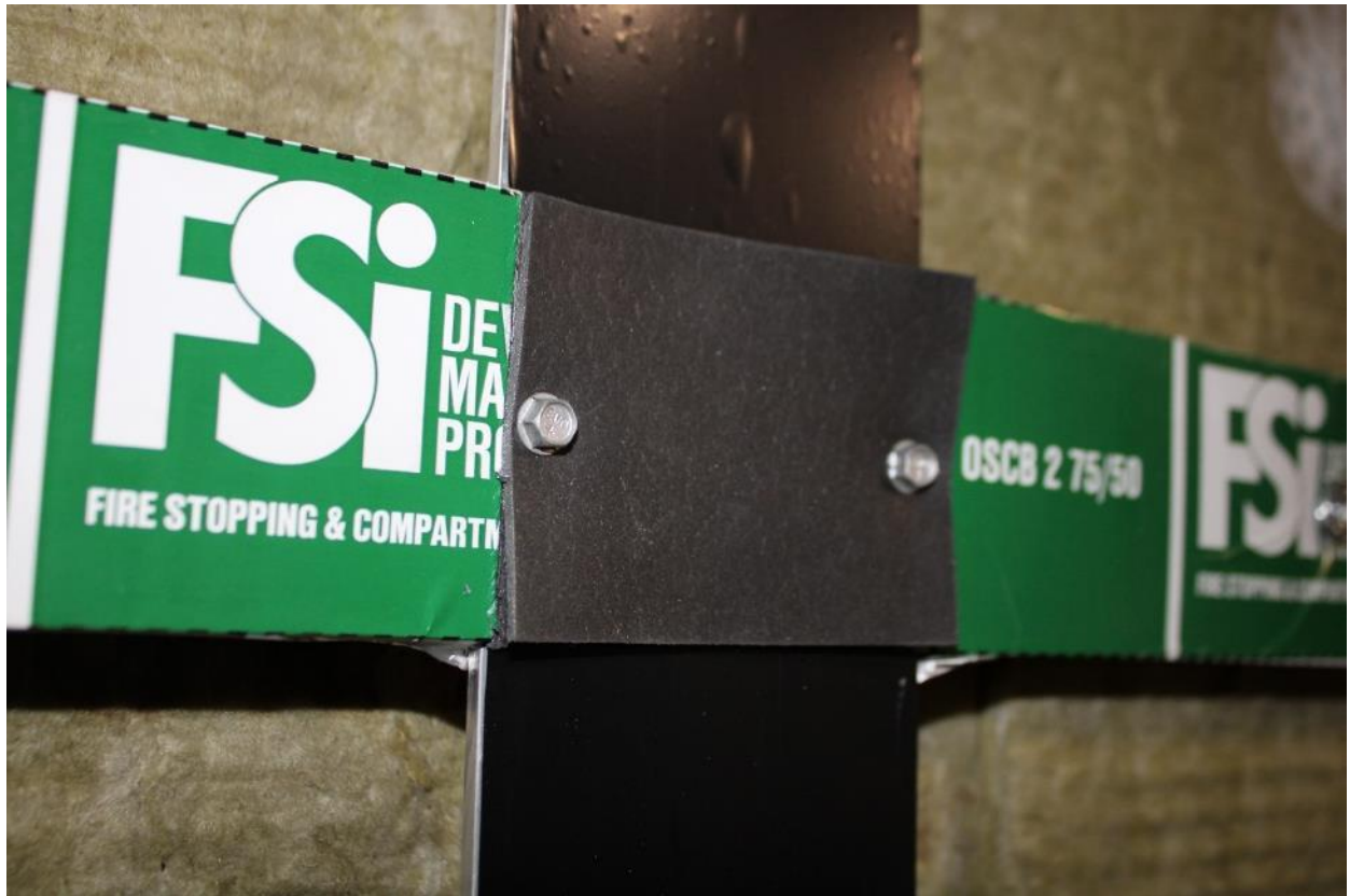
Figure 24. Intumescent strip applied to face of rail.
