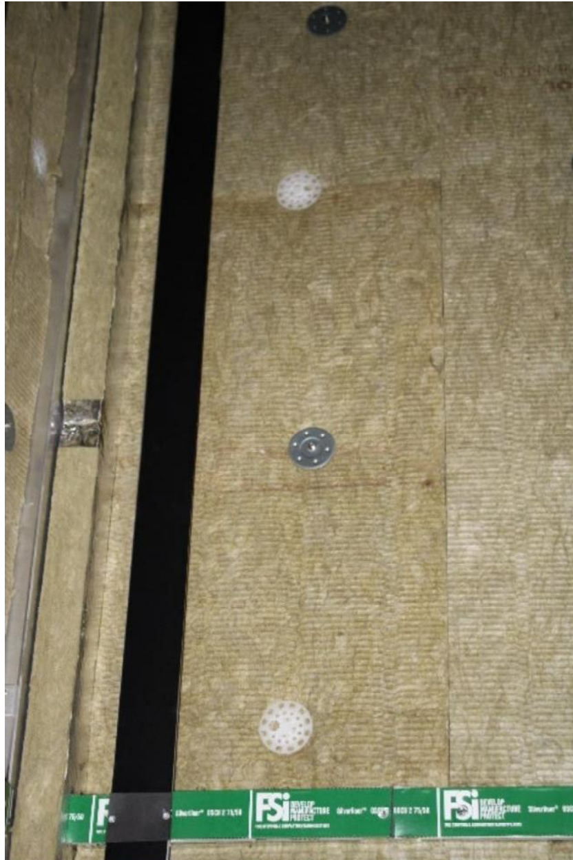
Figure 23. Close up of insulation fixing detail.
