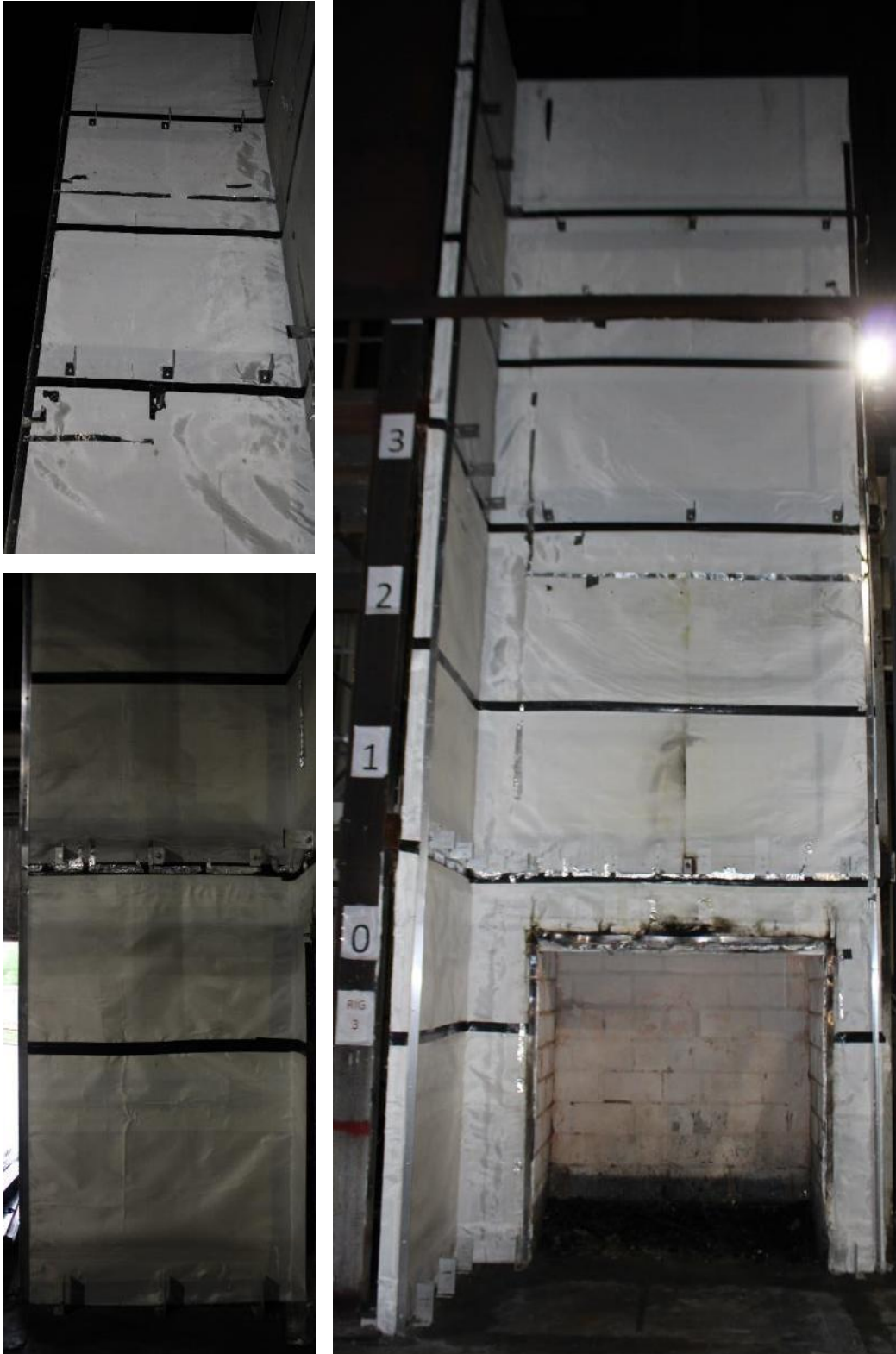
Figure 61. Full-height photograph of the breather membrane and aluminium brackets.
