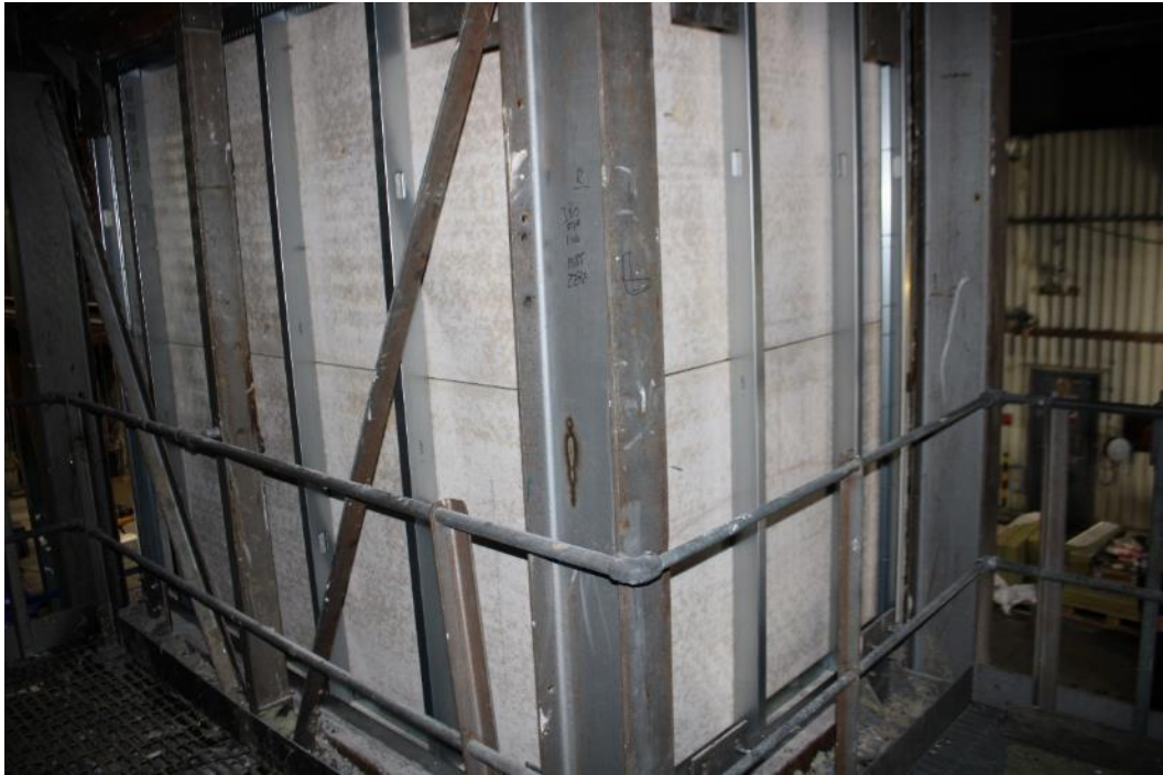
Figure 64. Sheathing board at rear of system at level 1.
