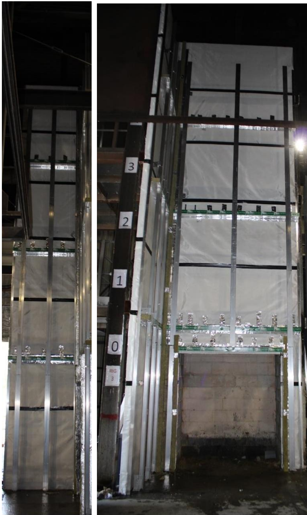
Figure 15. Installation of horizontal & vertical cavity barriers.
