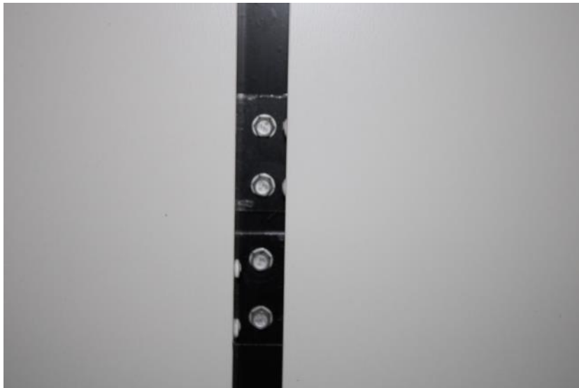
Figure 31. Panel fixings.
