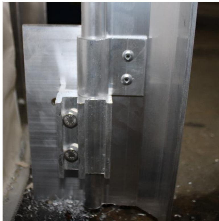
Figure 13. Aluminium dead load clip (Item 15).
