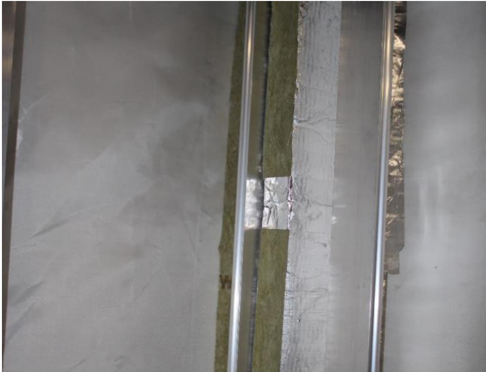
Figure 18. Vertical cavity barrier joint.
