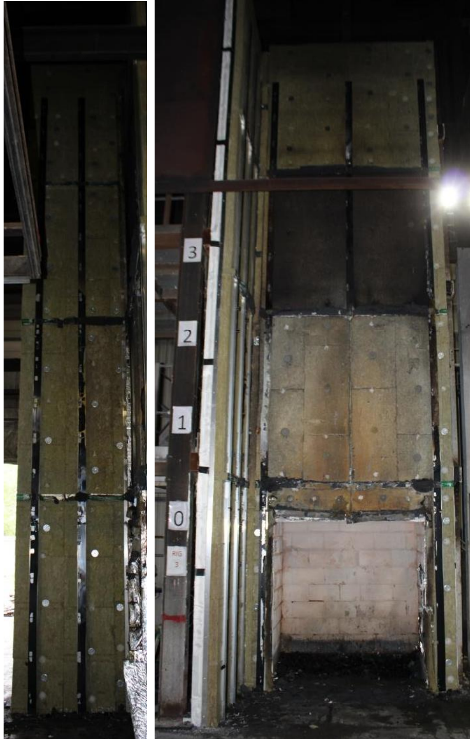
Figure 53. Full-height photograph following removal of panels.
