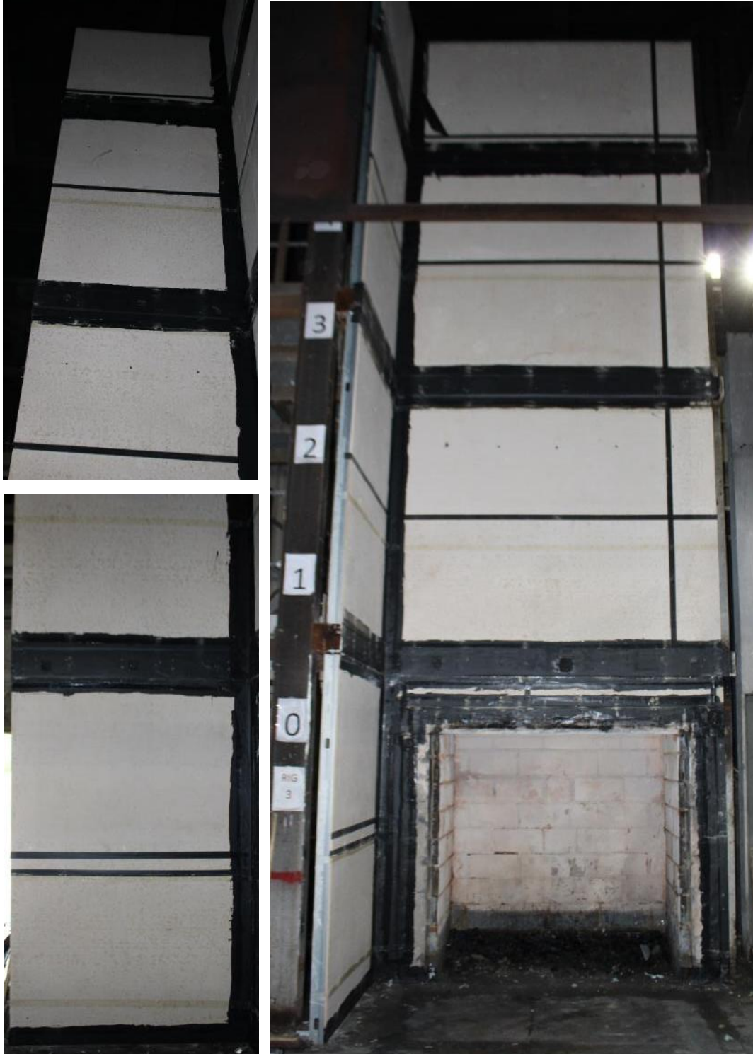
Figure 63. Full-height photograph of the sheathing board & EPDM membrane.
