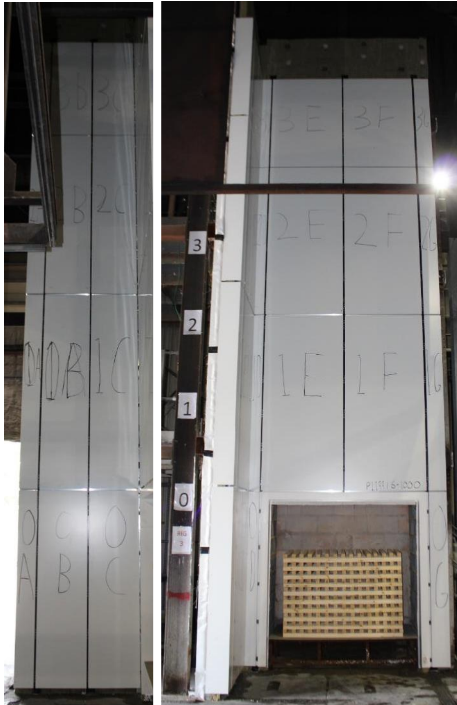
Figure 33. Completed installation prior to test.
