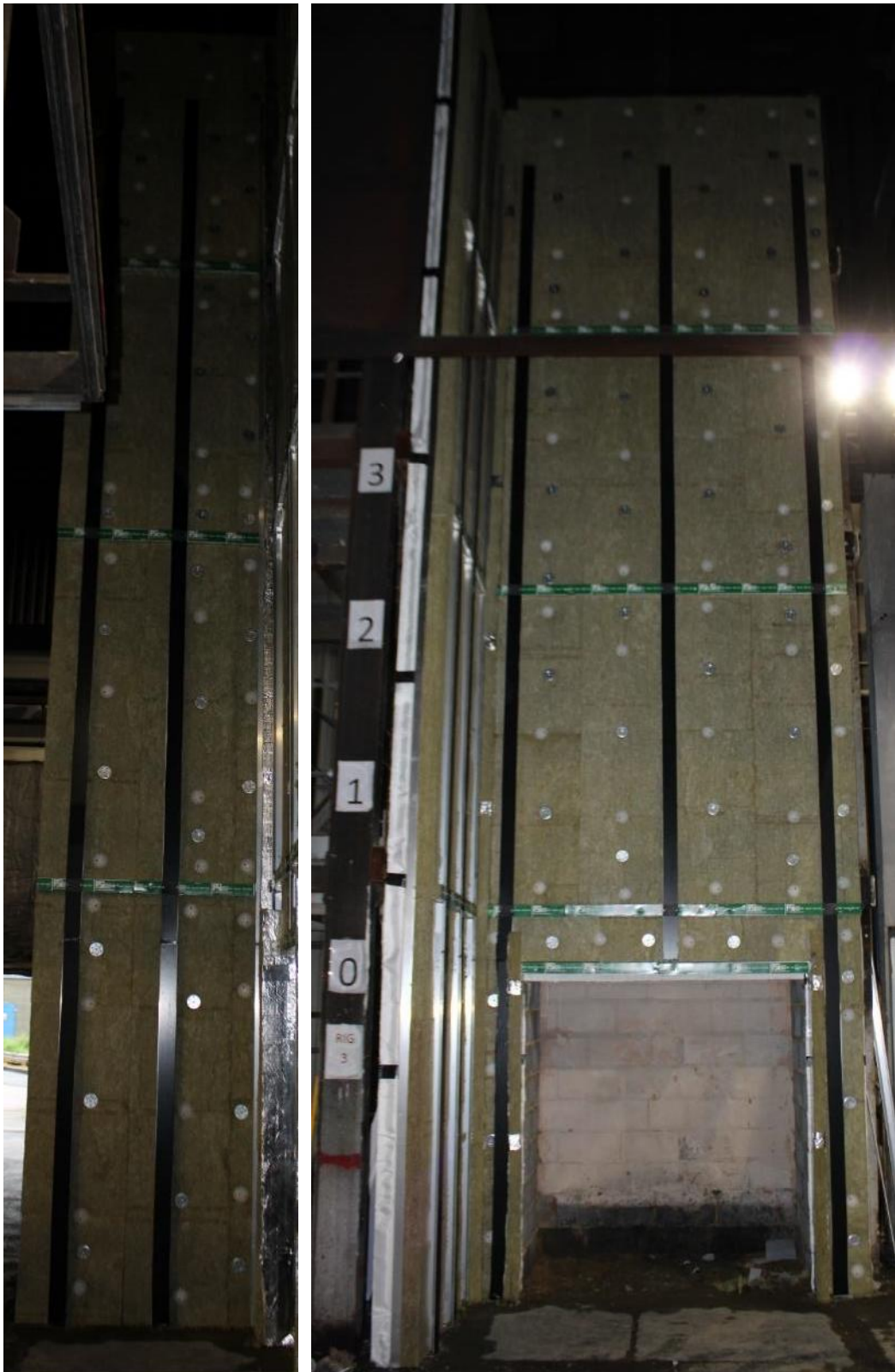
Figure 20. Installation of the insulation & and intumescent strip.
