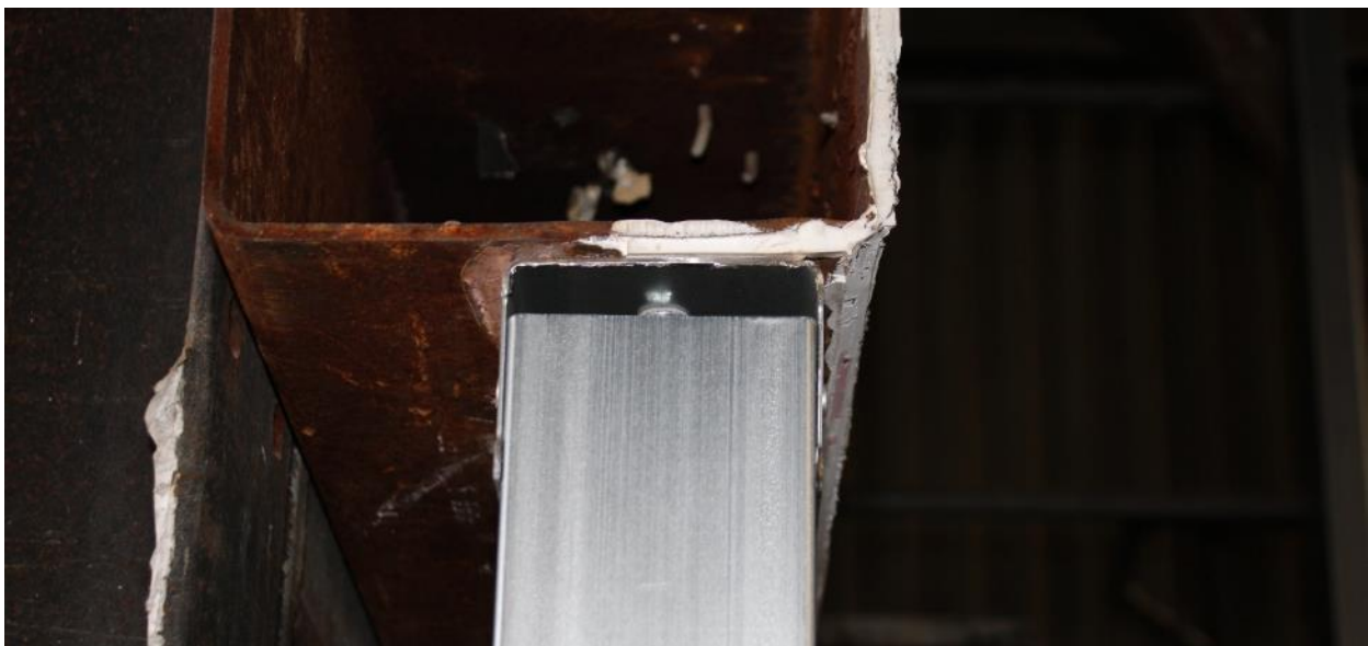
Figure 4. SFS location on the square hollow section (SHS).
