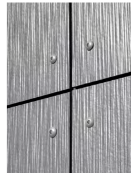
Hardie® Panel Rivet Fixing
