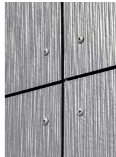
Hardie® Panel Screw Fixing
