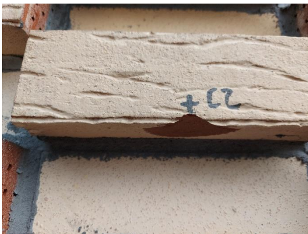
Showing damage caused following impact reference C2 on the orange zone
