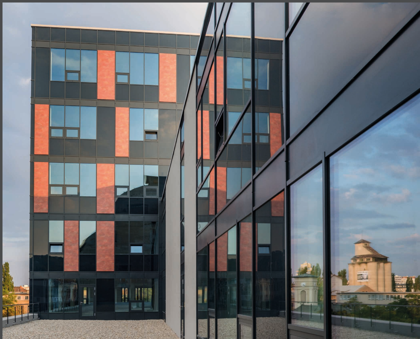
Stein 2 Office, Slovakia | Material: ALUCOBOND® PLUS vintage Coracero | Architect: Ateliér Ivan Kubík | Fabricator: ALUSTEEL | © Martin Viazanko
