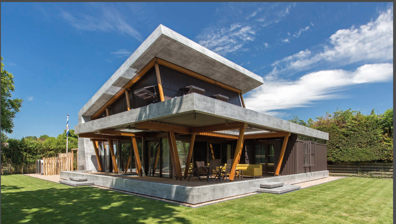
Holiday Home, the Netherlands | Material: ALUCOBOND® PLUS vintage Rough Concrete | Architect: Architekenburo TEN HOVE B.V. | Fabricator: MZAllpro | Installer: Cladding Partners B.V.
