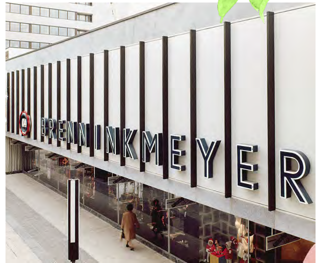
1969 Realisation of the first small façade project: C&A Brenninkmeyer in Leverkusen, Germany – very simple cladding with unformed panels
